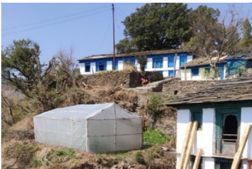
Figure 24. Polyhouse made from bamboo poles and plastic sheet.
