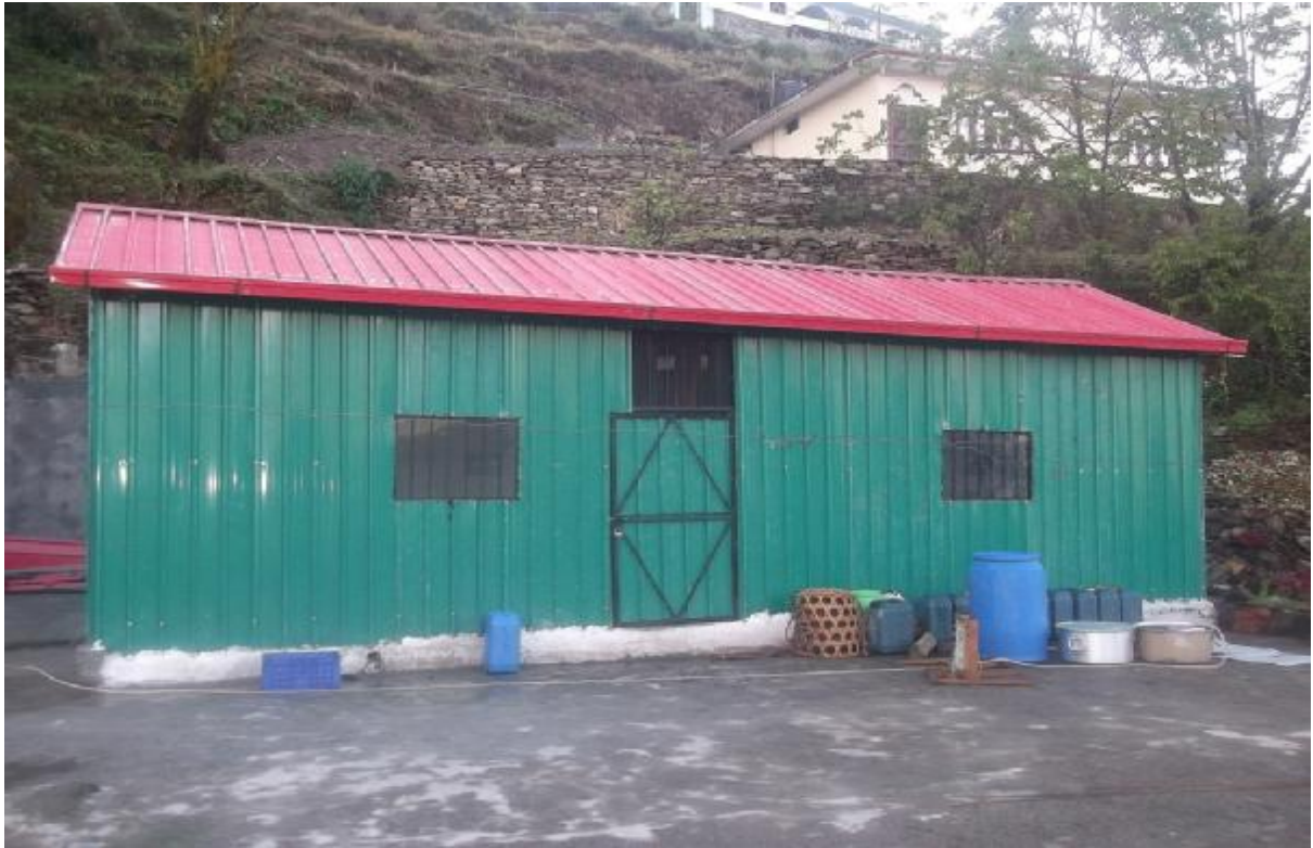
Newly constructed tin shed for fruit processing unit at Ukhimath
