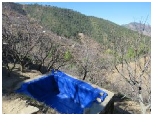
Figure 59. Old cracked, abandoned tanks were put into reuse by covering them by plastic sheets.
