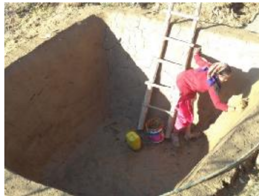
Figure 57. Before putting in the sheets, tanks were plastered by mud several times.
